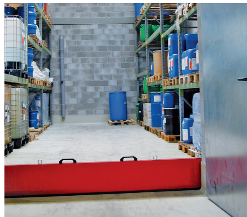
Spillage/fire fighting water retention (Photo source: Environment Office, Ct. TG)
