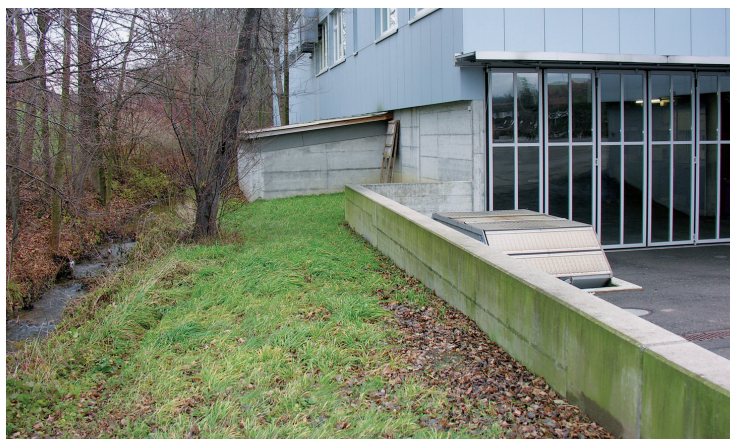
Flood protection for chemical stores (Photo source: Environment Office, Ct. TG)
